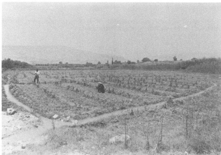
FIG. 91. Tertiary canals at Al-Mansheih taking water to cultivated fields and quaternary canals within the fields.
