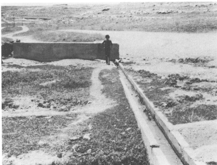
FIG. 81. A capped artesian well at Qualiba spring (near Irbid) with a concrete conduit for transporting its water.
